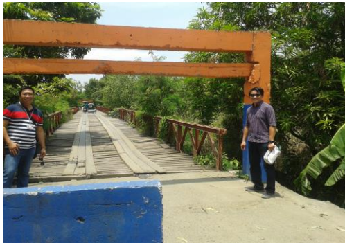
Fig. 1. The Abulalas & Carillo Bridge, Hagonoy, Bulacan.
